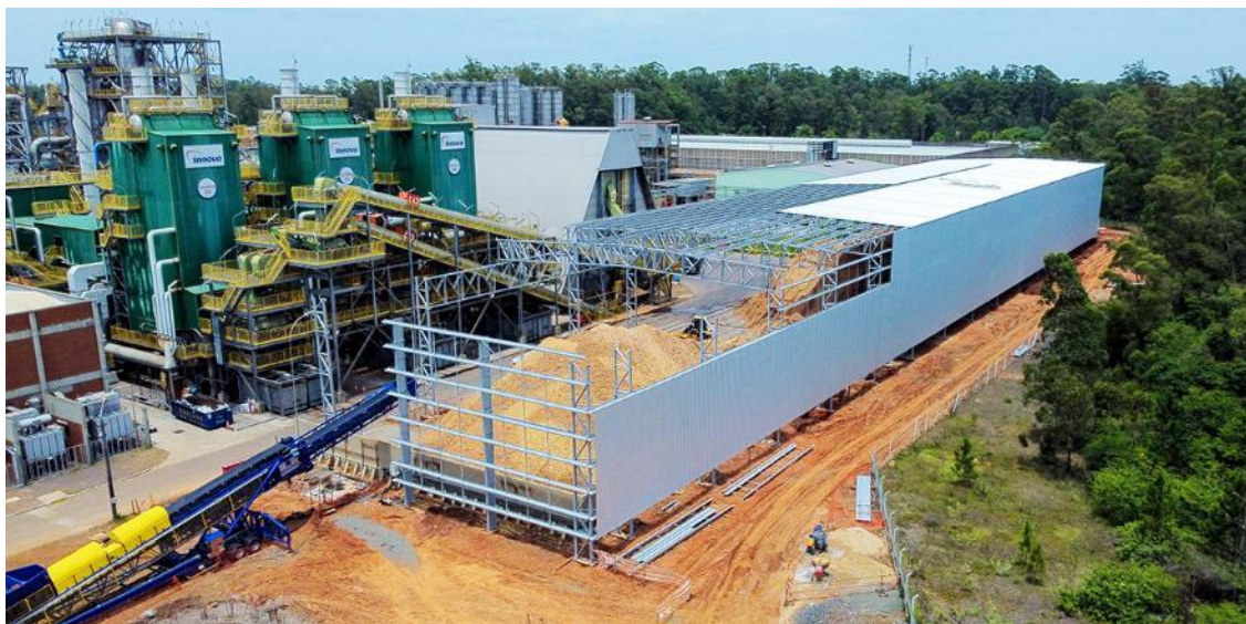
Plant II, Triunfo (RS), petrochemical: installation of the biomass yard warehouse
